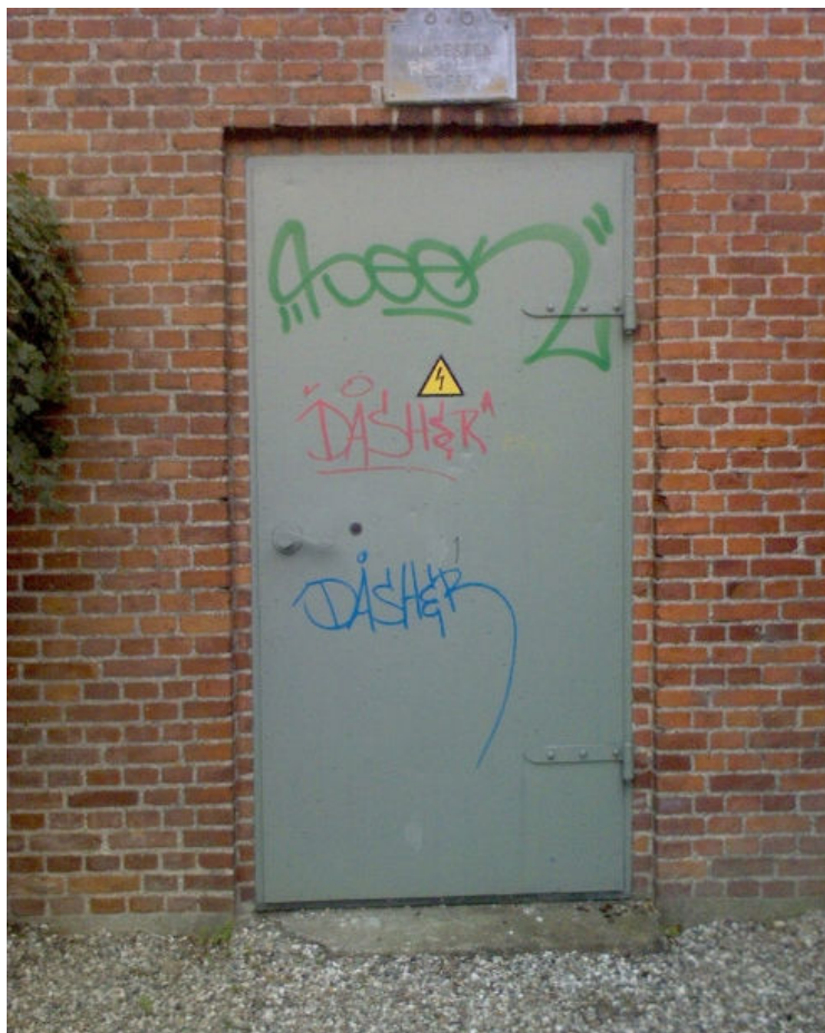
Hvidesten – transformatorstation. Foto poj
